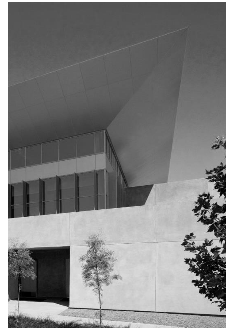
INVERTED MANSARD ROOF
